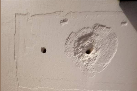
Patched wall surface showing previous fixings and uneven repair, revealing layers of interference.
